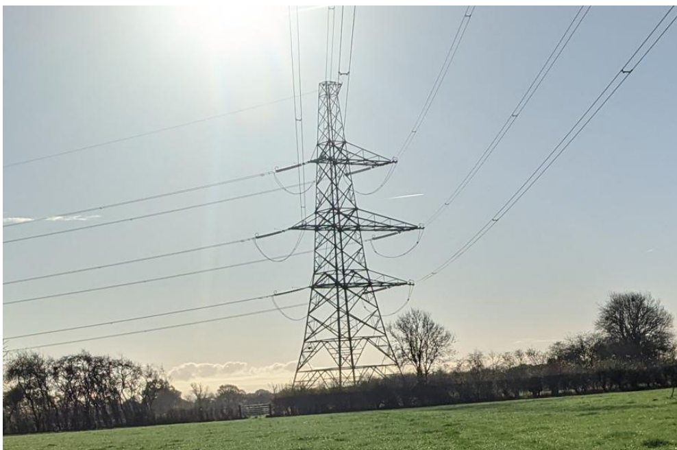
Image 4.16 Typical tension/angle lattice pylon 25
