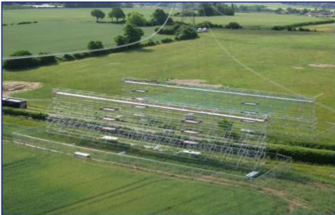
Image 4.11 Example of scaffold protecting a road crossing
