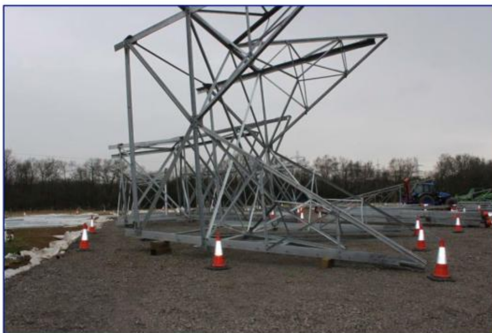
Image 4.5 Pylon steelwork preparation on the ground
