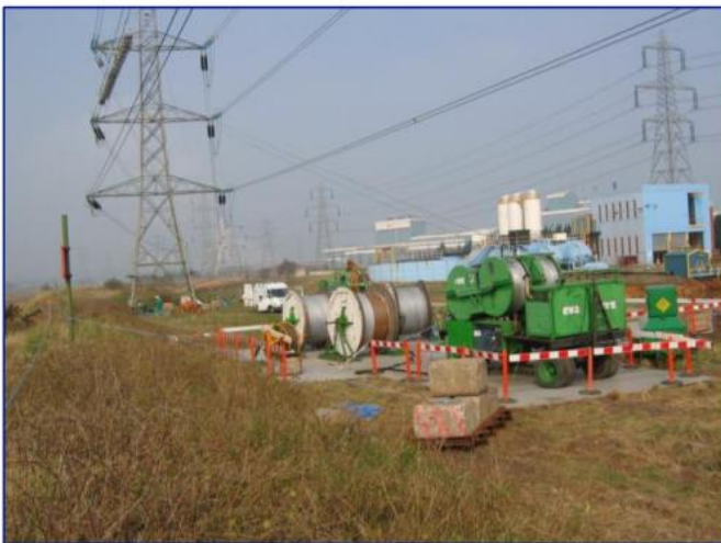
Image 4.7 Machinery associated with conductor pulling
